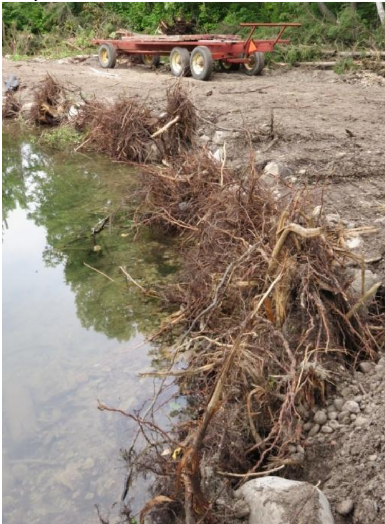
Shoreline before the undertaking of restoration efforts
